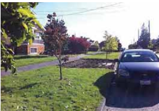
A recently-installed bioretention planter in a residential area.
