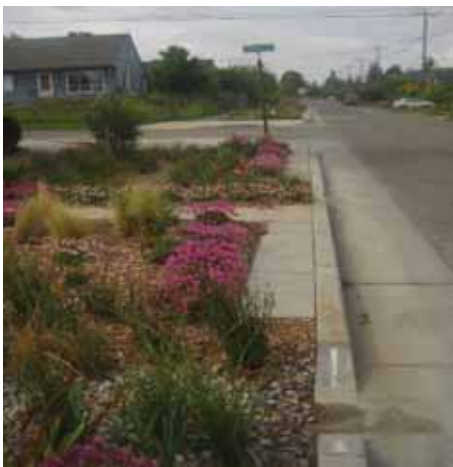
Both photos show infiltration cells used in a road diet.
