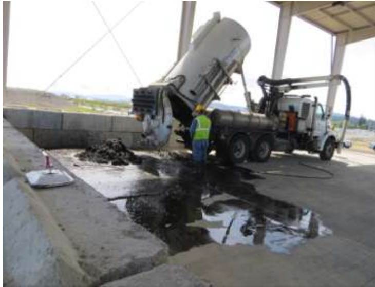
Fig-1 City of Spokane Decant Facility – vector unloading
