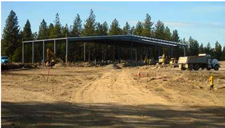
Fig-3 Spokane County Decant Facility – under construction
