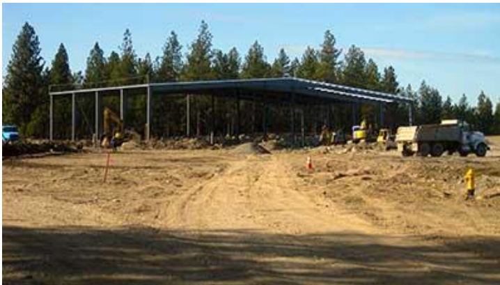
Fig-3 Spokane County Decant Facility – under construction
