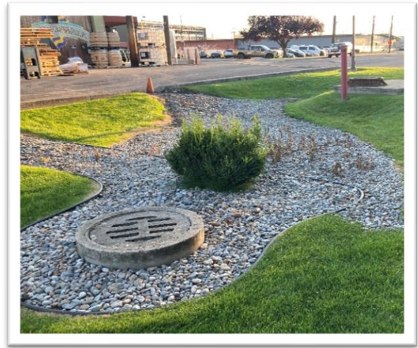
Figure 10. Drainage area at SW corner of 704 building.
