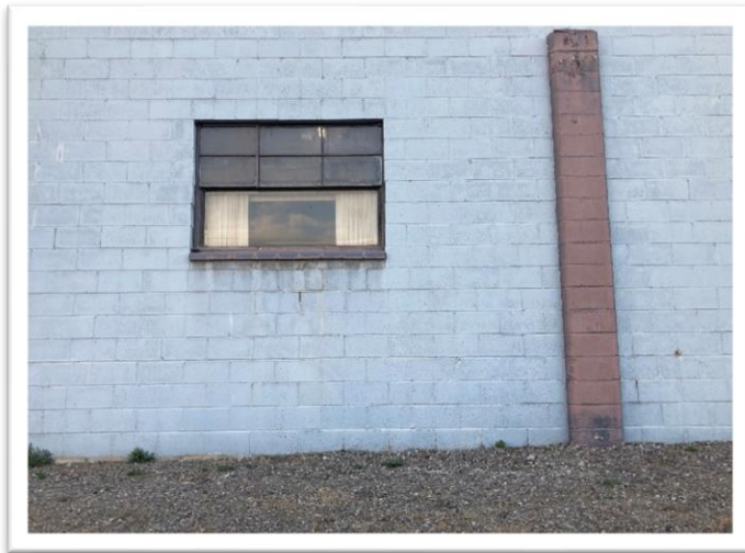
Figure 11. East face of 711 building.
