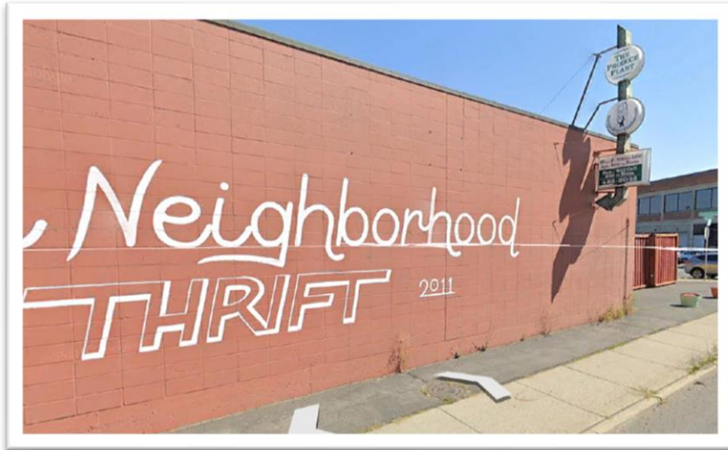
Figure 13. South side of 600/900 building
